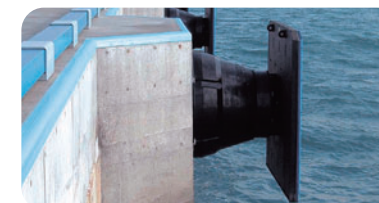
Civil Works and Marine Facilities
