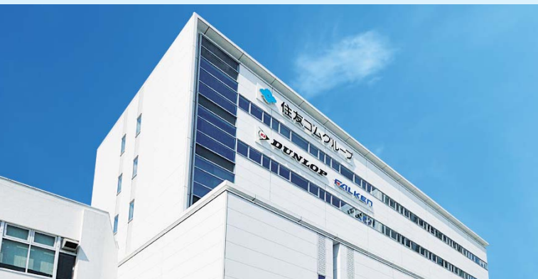
Tyre Technical Center Equipped with state-of-the-art testing and measuring machines, the Tyre Technical Center is the Group's main tire R&D facility.
