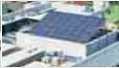
Rooftop solar panels
