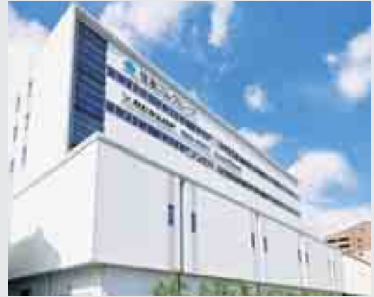
The Tyre Technical Center
