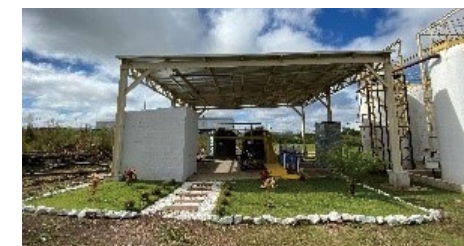
Wastewater recycling facilities (Brazil Factory)
