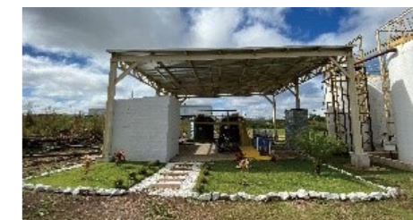
Wastewater recycling facilities (Brazil Factory)
