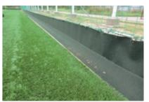
Barrier materials for use in the outer perimeter fences of artificial turf
