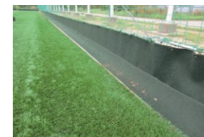
Barrier materials for use in the outer perimeter fences of artificial turf
