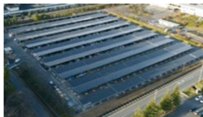
Solar power generators
